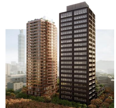
Daan District Office Building 5
