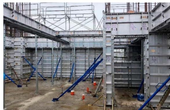
Assembly of the System Formwork for Sheng Lian Development's Tainan Ximen Complex – Life with Books & Garden Building Project
