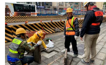
Sidewalk Repair Operations
