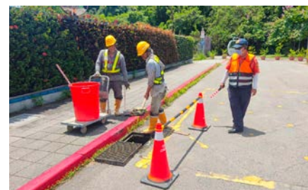
Drainage Ditch Dredging Operations
