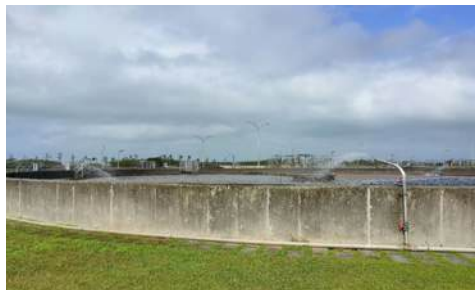
De-foaming Water from Secondary Clarifier
