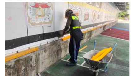
Repairing the Anti-Collision Strip on the Elementary School Playground
