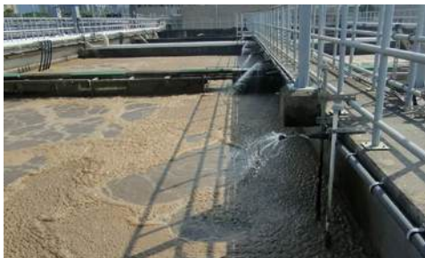
De-foaming Water from Aeration Tank
