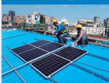
Installation of Solar Energy Equipment
