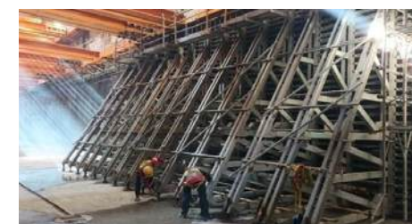
System Formwork Assembly
